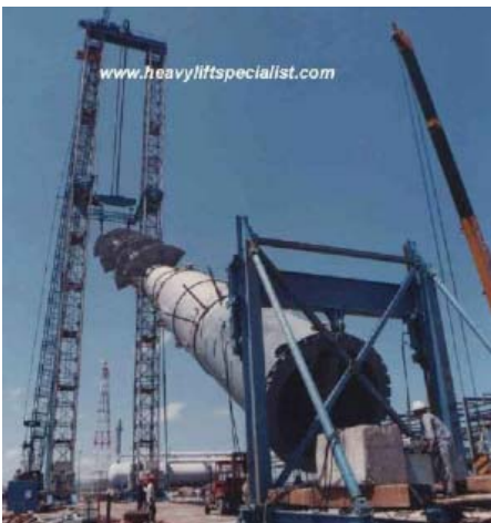
Erection of a 220 Tons column with an unguided lift gantry in Kerteh Malaysia, project was carried out in close co-operation with freight forwarder Kontena Nasional
