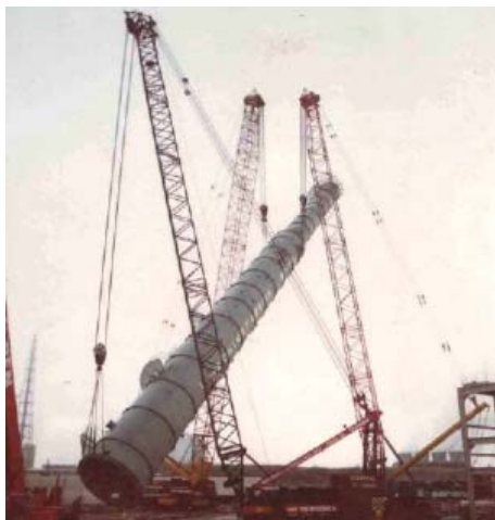
Lifting of a 330 tons CO2 tower at NSM in Sluiskil
