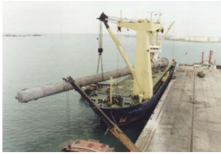
Shipment and Transport of Heavy Columns for TPI Refinery Rayong, Thailand
